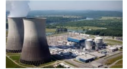
For a nuclear facility
